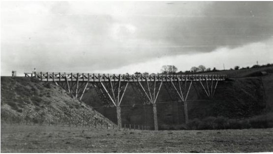
A rare photograph of Ringwell viaduct. It was demolished and an embankment built when the Carnon Valley wooden viaduct was replaced in 1930s with an impressive granite and concrete structure
