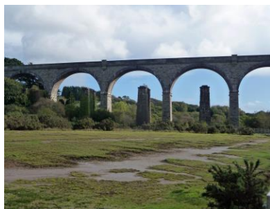
View of Carnon Valley viaduct nowadays with the pillars of the original one seen behind (T. Dundon)
