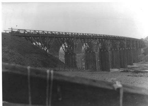
A clear view of the intricate fan-shaped supports of the original Carnon Valley viaduct designed by Brunel. The modern 1930's version can be seen behind.
